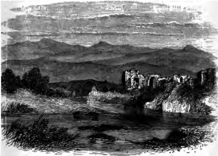
BRIDGE OVER JORDAN.
